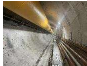
TBM tunnel 2 x 1.8 km twin tube 6.24m int. diameter
