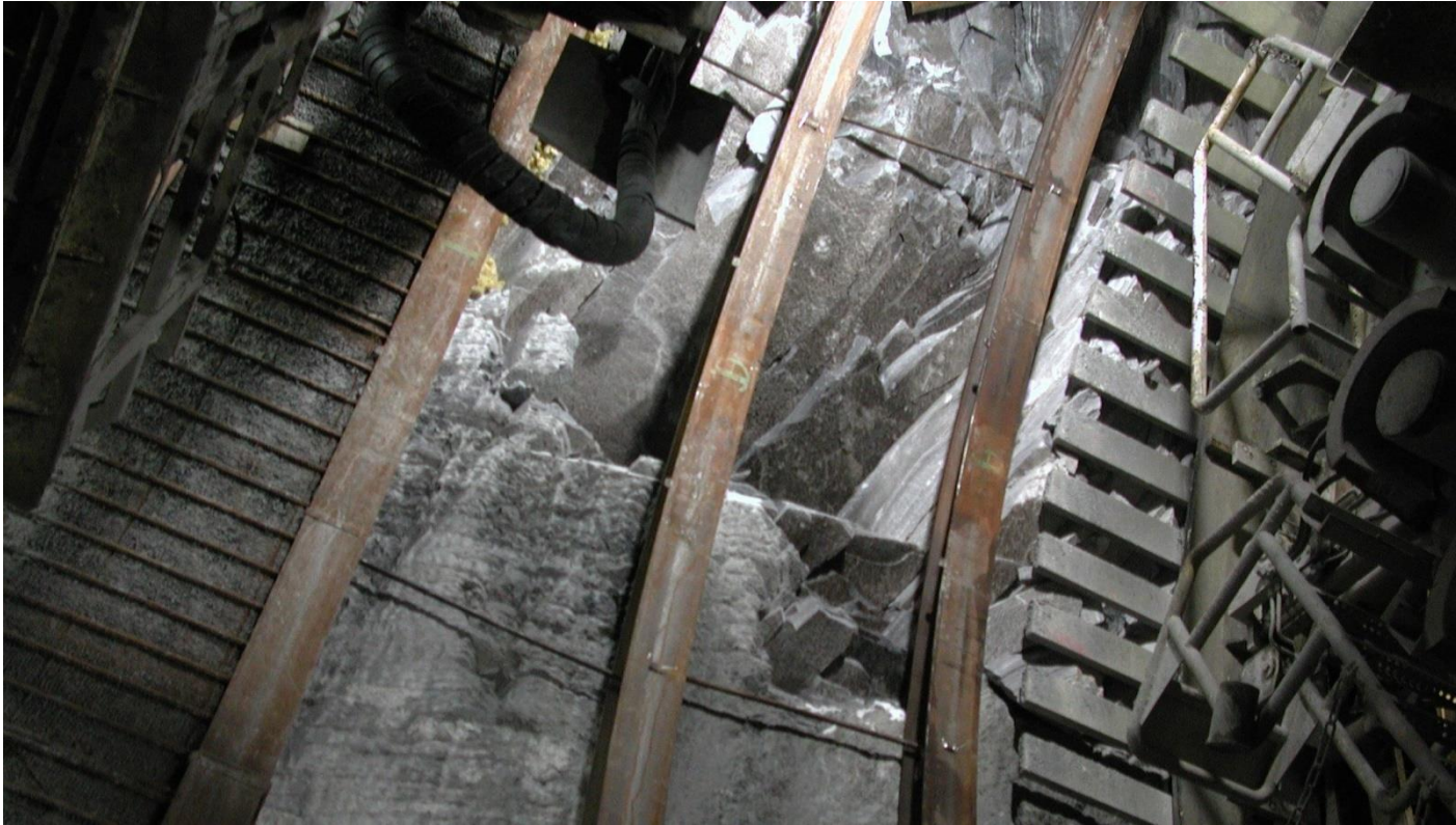
Localized brittle failure of intact rock and movement of blocks.
