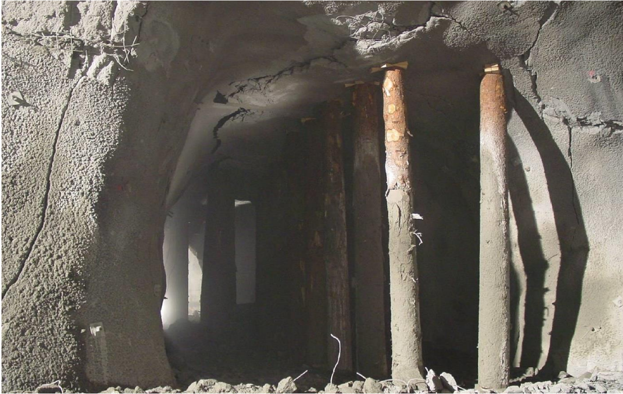
Squeezing and swelling rocks. Elastic/plastic continuum.
