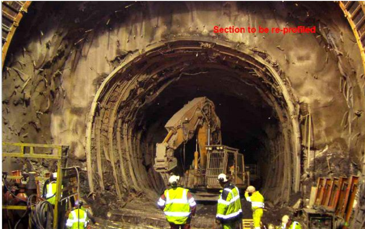
Squeezing and swelling rocks. Elastic/plastic continuum.
